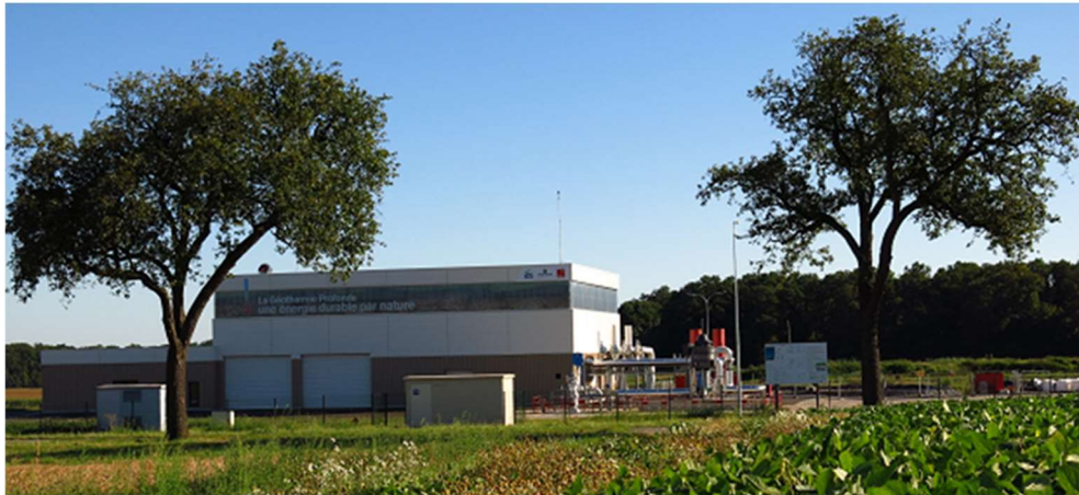
Figure 1 View of the Rittershoffen geothermal heat plant (ES-Géothermie)
