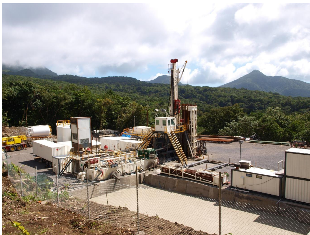
Figure 8: Drillrig Sleipnir from Iceland drilling during drilling of well WW-3 at Laudat Dominica in 2012. The photo shows a 1300 m 3 "sump" system in the foreground. Photo: Sigurður S. Jónsson, ÍSOR.
