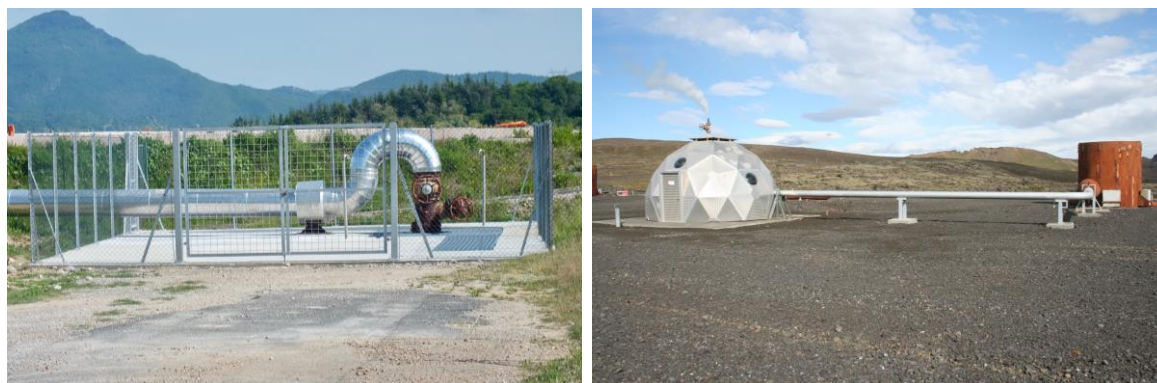
Figure 5: Left: a wellhead in Italy. Right: Enclosed wellhead (left) at Hellisheidi power plant in Iceland, connected to a muffler (right). Photo: A. Manzella (left), Mannvit, 2013 (right).
