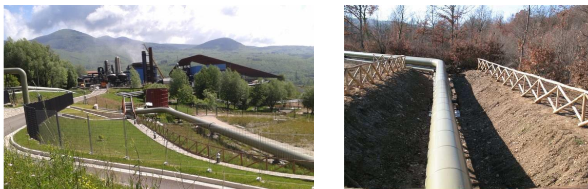
Figure 3: Examples from Italy. Left: Bagnore 3 power plant in Italy, planted trees to reduce visibility of infrastructures. Right: trench for pipeline. Photo: Enel Green Power.
